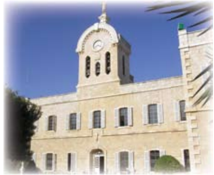
De La Salle Hall at Bethlehem University was built in the year 1893 to house the Christian Brothers elementary school known as Freres School. In 1973 Freres School moved to a different location and Bethlehem University was founded by three Brothers from the U.S.
